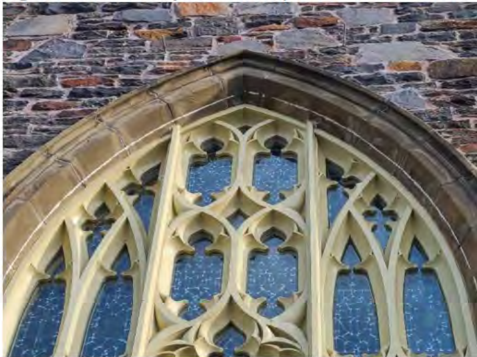
Figure 35j: First Baptist Church, 1300 Oxford Street – top of west side window showing wall efflorescence and deterioration at mortar joints
