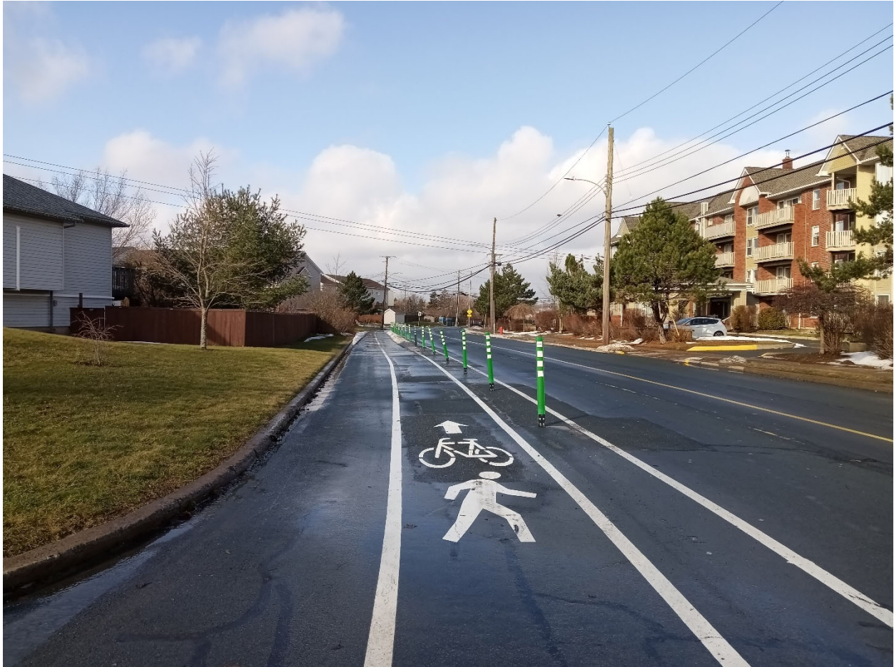
Travel lanes narrowed using paint and flexible bollards. Remaining lane space was converted into a bi-directional multi-use pathway
