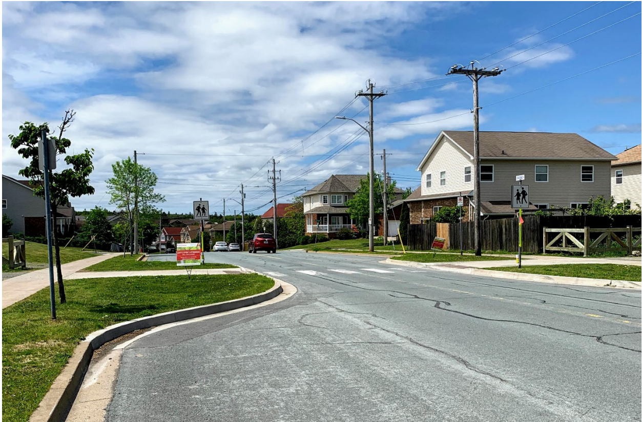
Curb extension at marked crosswalk
