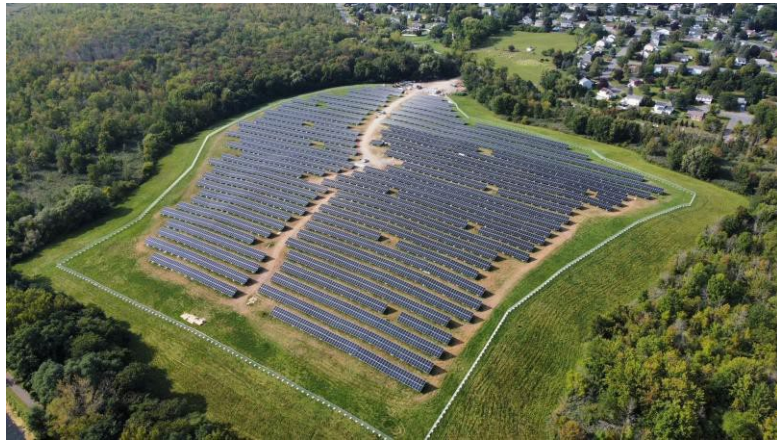
Illustration of solar farm built by SolarBank
