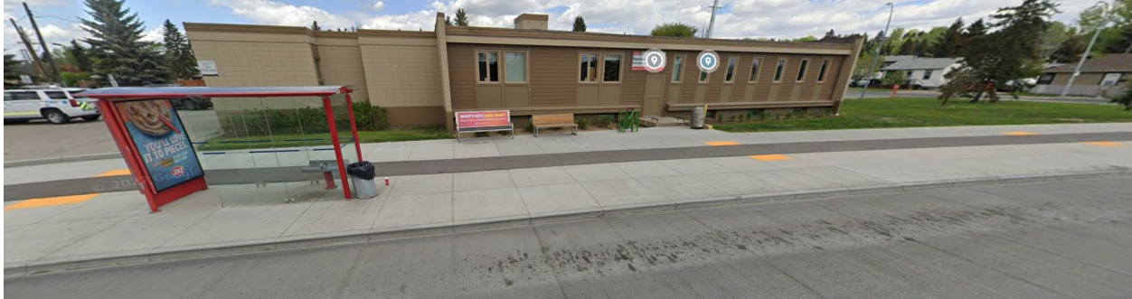
Figure 18: Calgary site at Home Road / Bowness Road (north corner)
