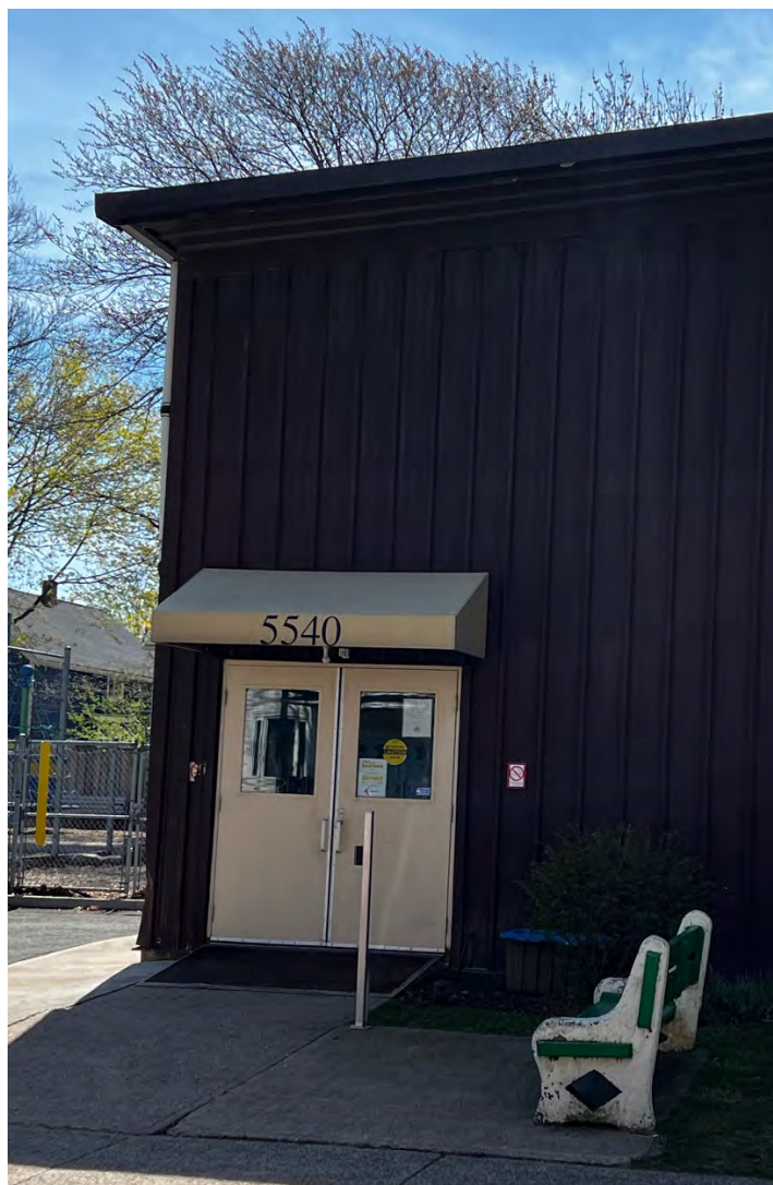
Figure 40: Paired entry doors, 5540 Russell Street
