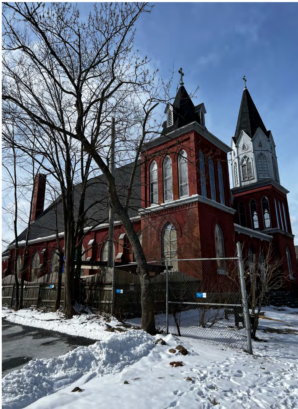
Figure 30b: Front and south side of 5522 Russell Street
