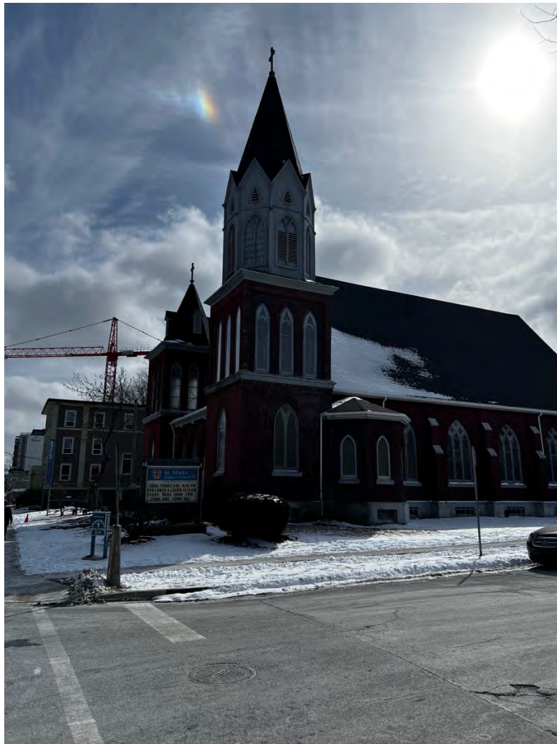
Figure 29a: Context of St. Mark's Church, 5522 Russell Street (seen from corner looking south along Gottingen Street)
