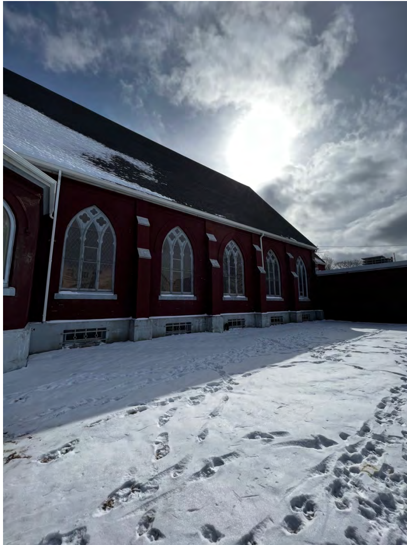
Figure 41l: St. Mark's Church, 5522 Russell Street (north side wall)
