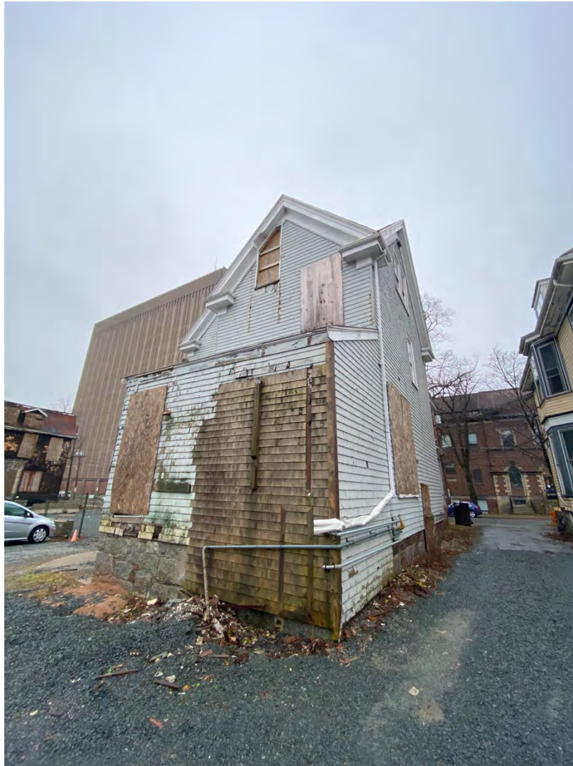
Figure 23b: Shed roof addition at the rear of 5963 College Street
