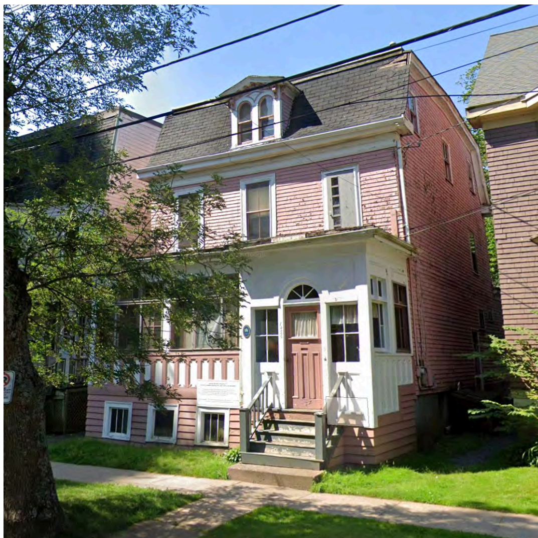
Figure 31: 1456 Carlton Street, in 2019, prior to extensive exterior alterations Source: Google Streetview
