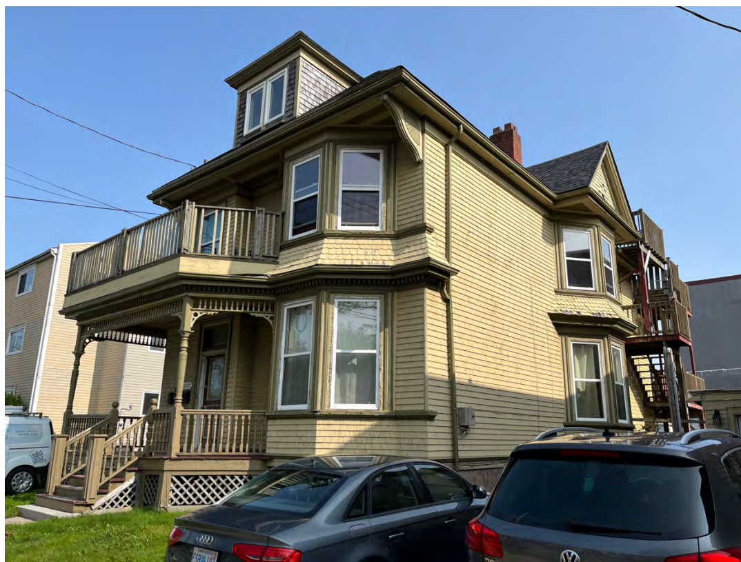
Figure 29a: 1377 Robie Street, front and south side
