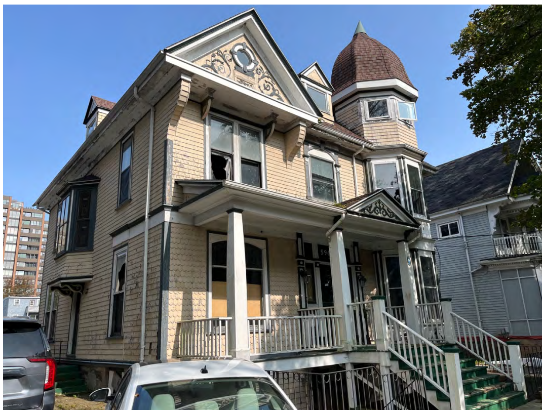
Figure 27a: Gold Cure Institute, 5969 College Street – front and west side
