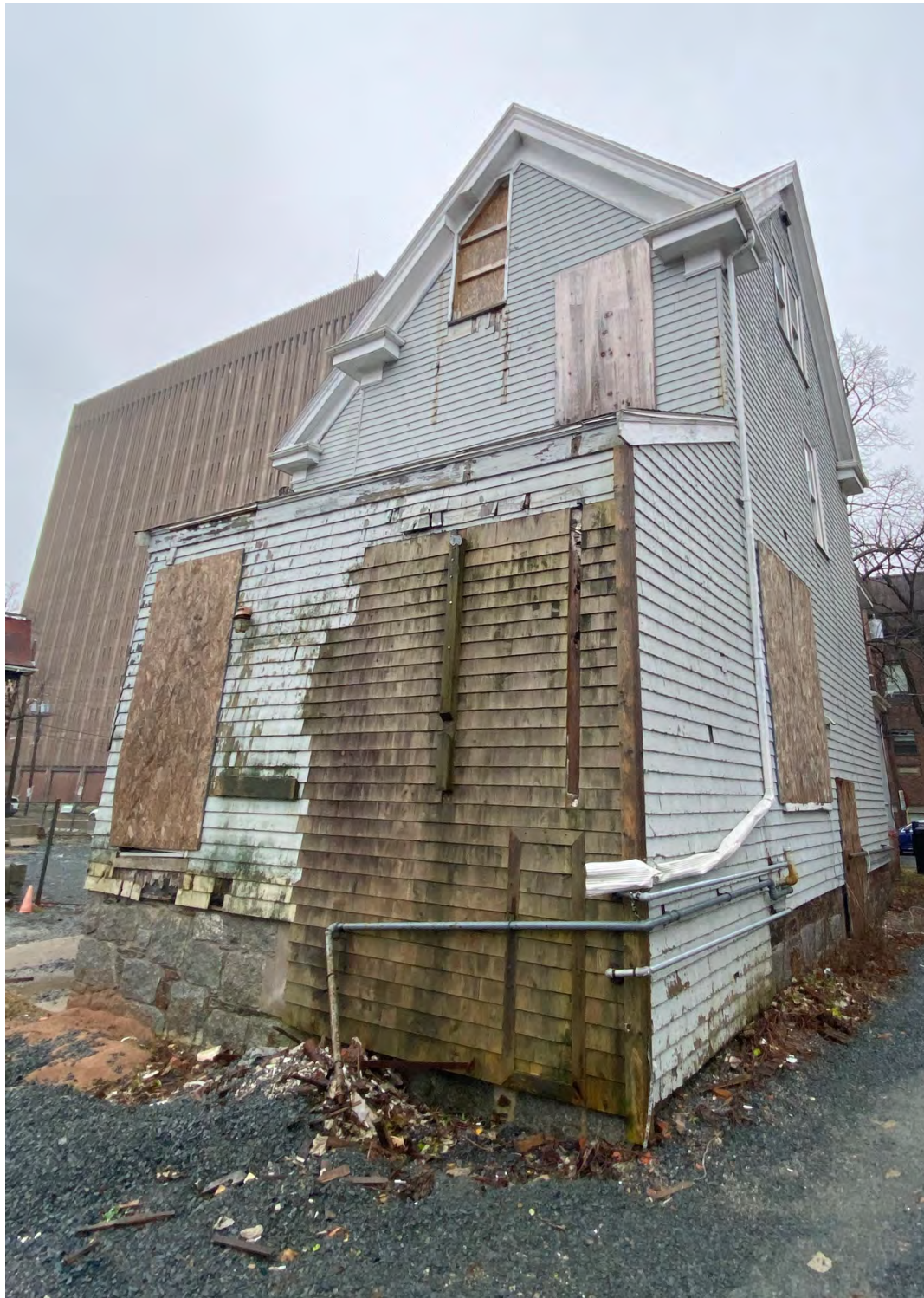
Figure 35d: MacCoy Residence, 5963 College Street (Rear)
