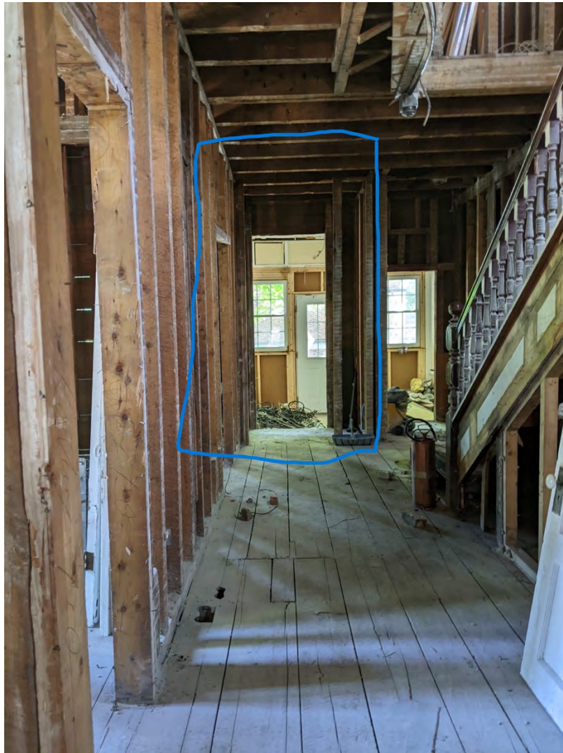
Figure 21d: Interior view of front door and window openings behind enclosed porch, 5963 College Street
