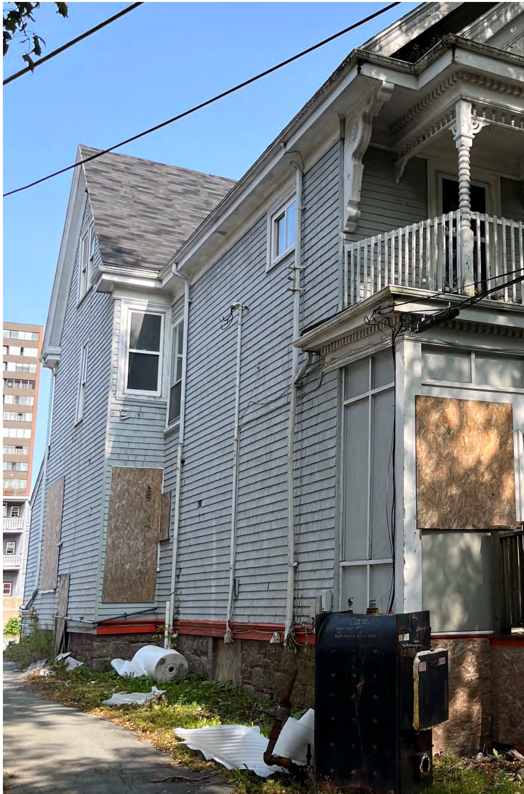
Figure 35c: MacCoy Residence, 5963 College Street (East side)
