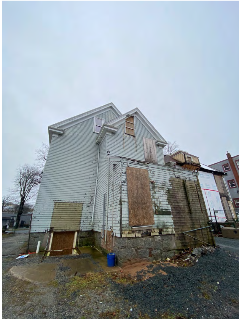
Figure 21c: Rear of 5963 College Street
