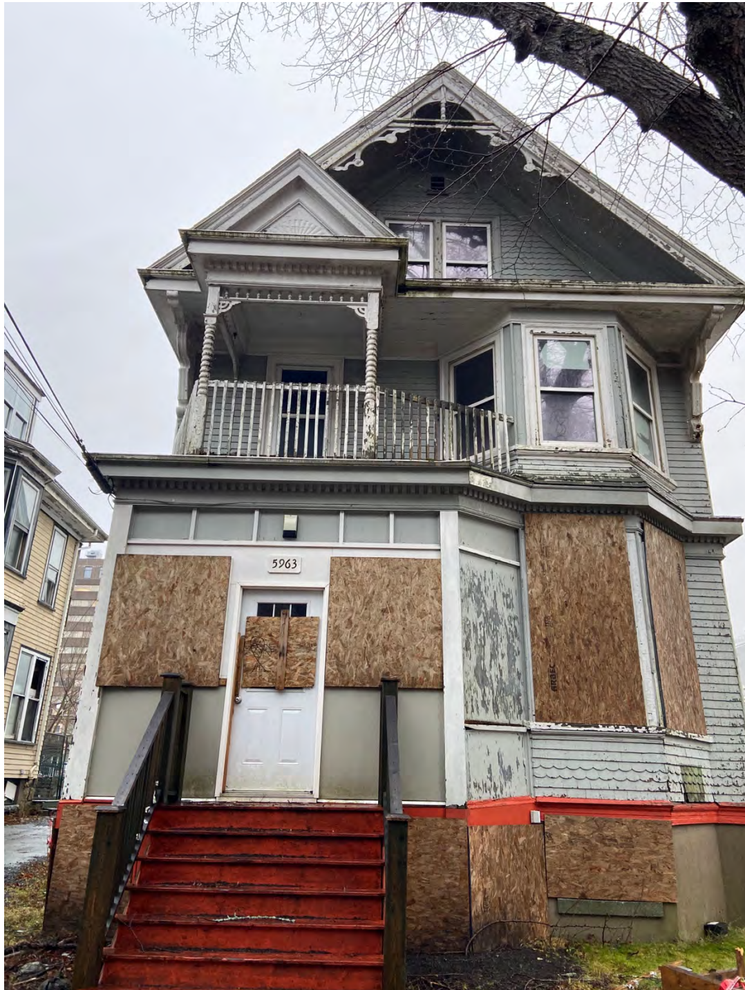
Figure 35a: MacCoy Residence, 5963 College Street (Front)
