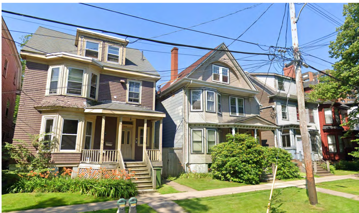
Figure 10: Registered houses immediately north of subject site on Carlton Street: early Victorian houses (left and far right) with a 1906 Edwardian house (centre right)
