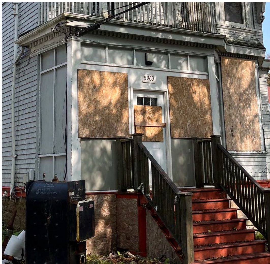
Figure 23a: Front porch enclosure of 5963 College Street
