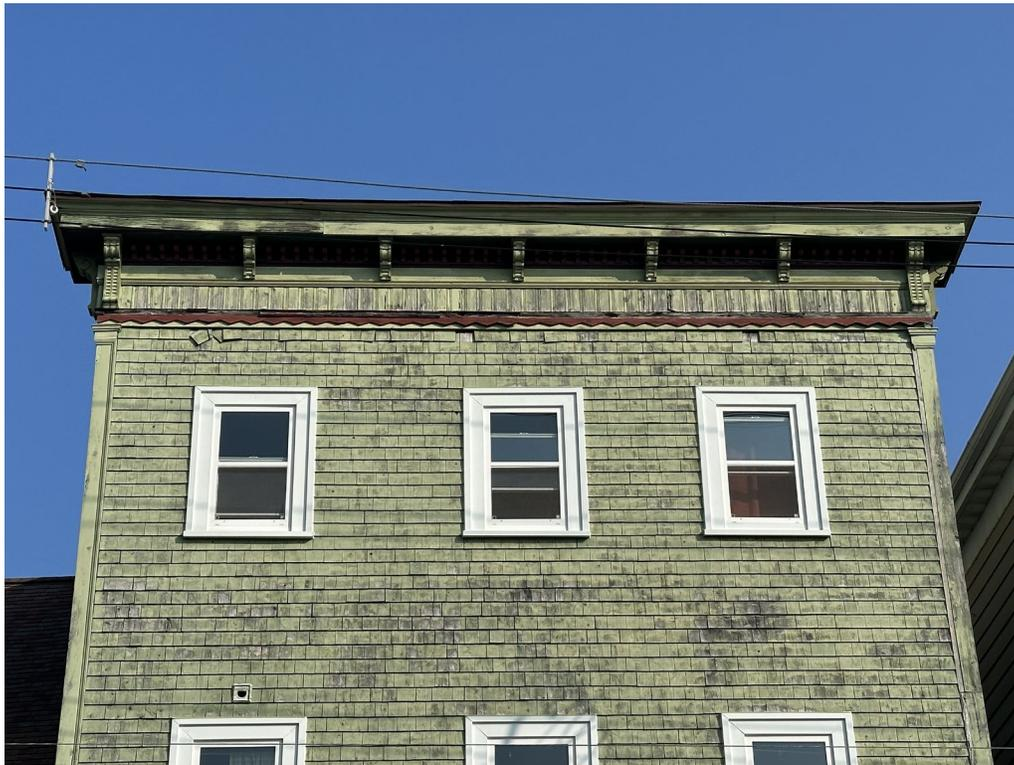
Figure 13: Decorative bracketed cornice and corner boards on the south elevation of 5561 Cogswell Street. The prominent cornice, brackets and decorative trim is the work of the late Hal Forbes (September 2023)
