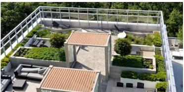
Image 9: Examples of Tall Guardrails for Wind Control
