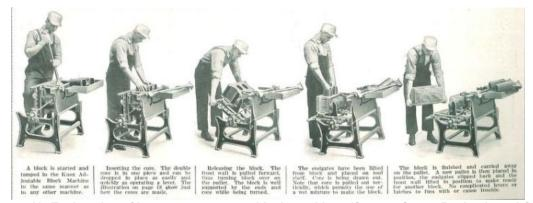
Figure 13: Explanation of how to use concrete block machines (Source: Sears, Roebuck, and Co.)
