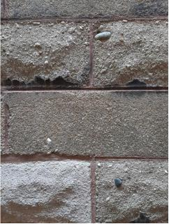
Figure 20: Concrete block cladding of 1741-1743 Henry Street. Note pieces of shell and aggregate incorporated into some of the blocks (Staff Photo, 19 May 2023)
