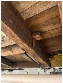
Figure 13: Mortise and tenon construction as visible from the basement of 1206 Robie Street (Source: **Property Owner)**
