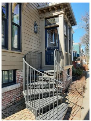
Figure 22: Curved staircase leading to the exterior wood glazed door with transom above on the storm porch.
