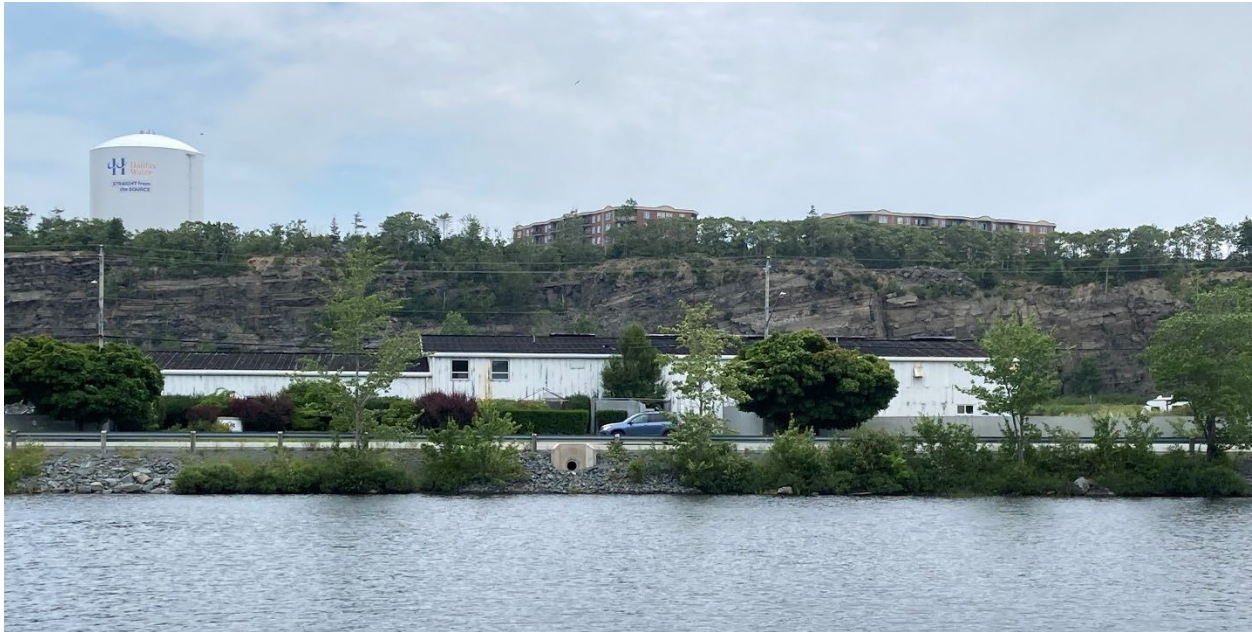
Figure 2: Riprap shoreline with partial vegetative cover along Kearney Lake Road.
