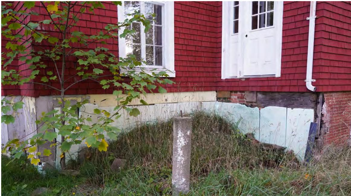
Figure 25: Detail view of foundation damage to northwestern corner of 144 Pleasant Street (October 19, 2021)
