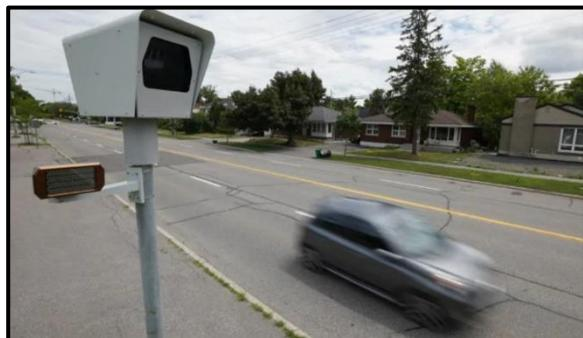
Fixed speed enforcement camera systems are installed roadside, similar to the manner in which red light camera systems are installed. Deployment requires installation of a pole for the camera housing and flash as well as a power connection. There is not a great deal of flexibility in terms of changing locations of enforcement with this type of system. Some
