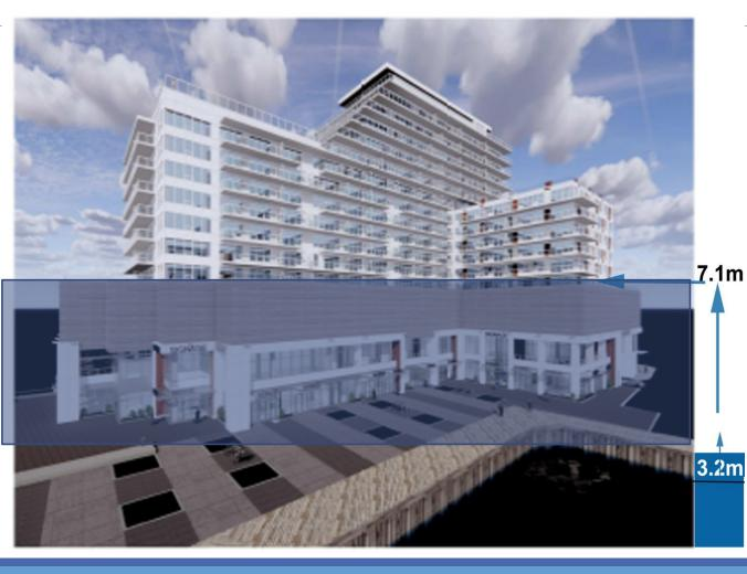
The model shows 1)3.2m setup used in Cunard plan versus 2) potential worst-case flood at a storm tide when Greenland melts
