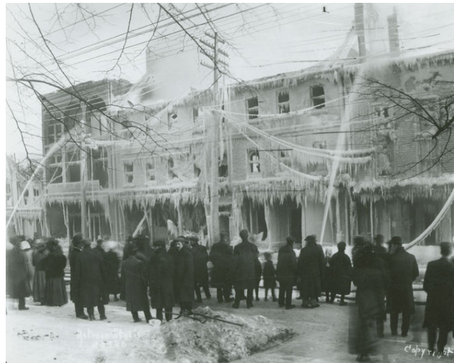
Fig. 4 1912 Barrington Street, looking east
