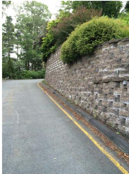
Photo 3: Retaining wall around bedrock outcrop.
