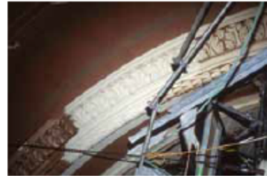
When restoring decorative plaster in the Walker Theatre in Winnipeg, moulds were made of existing plaster elements. The deteriorated plaster was then patched and repaired using the moulds to match the original.
