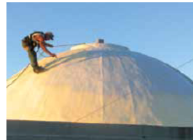
The dome of Melville City Hall was originally an uninsulated, painted-metal covering that caused persistent condensation problems. Applying insulating polyurethane foam with aluminized coating was a cost-effective solution that was compatible with the historic metallic look of the dome. If a more elaborate solution is contemplated in the future, the polyurethane could be removed.
