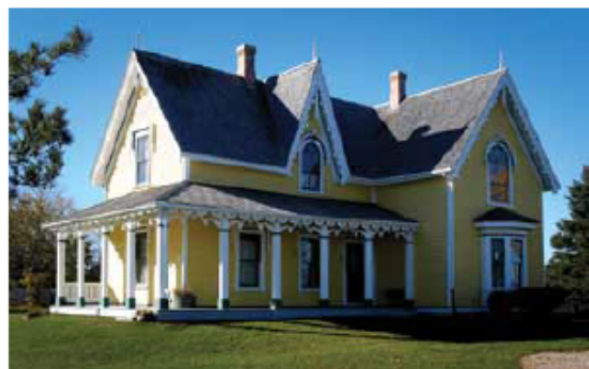
Based on documentary evidence, including an 1880 engraving, the original fenestration of the Bideford Parsonage Museum in P.E.I. was restored and roof finials replaced.
