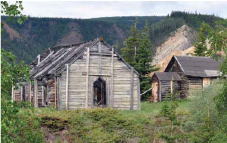
These buildings, along with others at St. Luke's Anglican Rectory and Church in the Yukon, were temporarily stabilized using a variety of measures including adding sandwich bracing, cable bracing, heavy frames, roll roofing, and covering door and window openings in order to keep out snow and rain. Stabilization allows the structures to be adequately researched and their eventual restoration to be planned.
