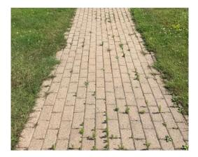
Figure 6 - Permeable pavers in Dartmouth; water can infiltrate between the blocks to a gravel bed below.
