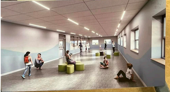
The renovations have started for the East Dartmouth Community Centre!
