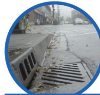
Storm Drains (Catchbasins)
