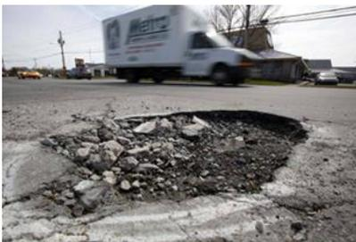
**Potholes** are caused when the asphalt on the surface of a road has deteriorated from the top,
