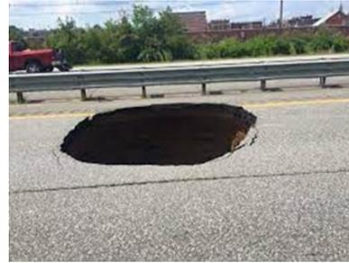
**Sinkholes** are caused by erosion from underneath, and when you look into the hole you cannot see any
