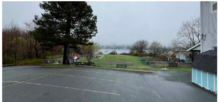
Fig. 6 The centre's parking lot defines much of the park's frontage, with the park itself recessed below.
