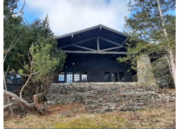
Arts and Crafts Style residence at 10 Kirk Road (March 2023)
