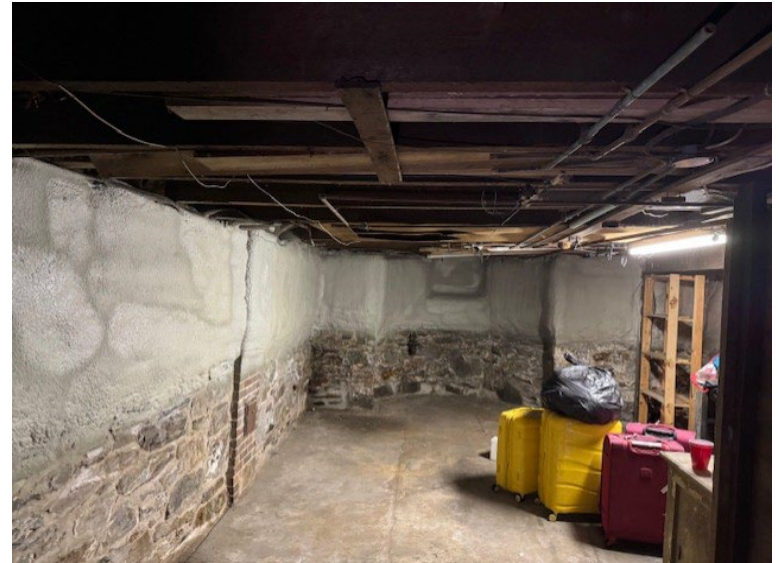
Interior foundation and framing
