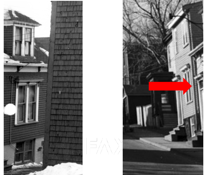
1960s Photo shows the changes of the dormer roof, window details and door transom
