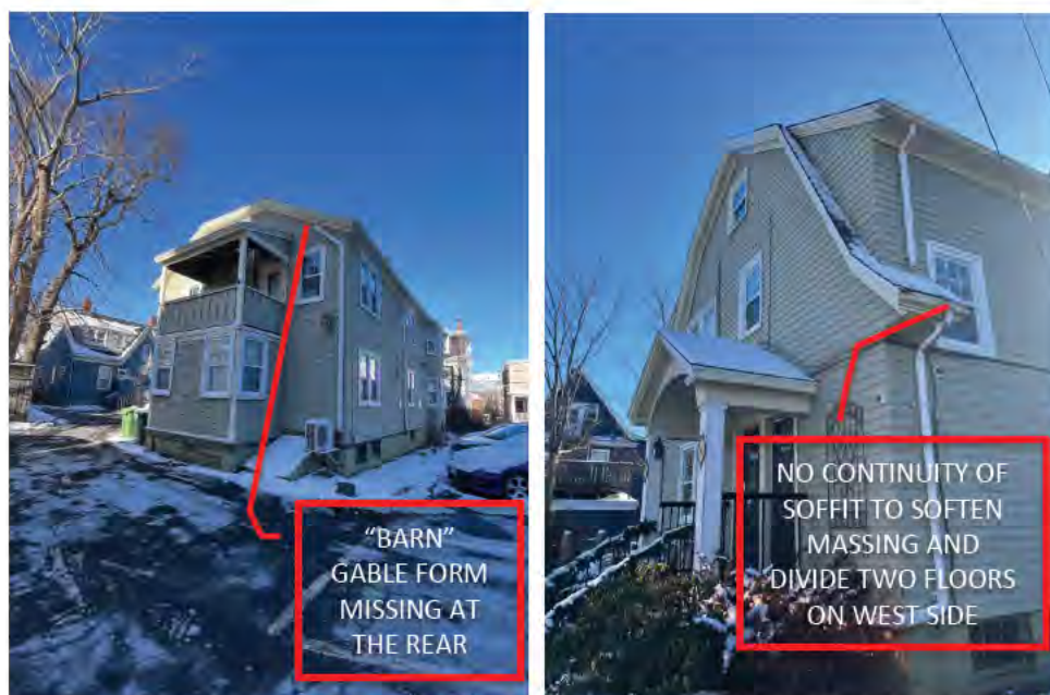
Figure 36c: Front and rear components of 43-45 Dundas Street that detract from the style and overall design of a Dutch Colonial Revival house.
