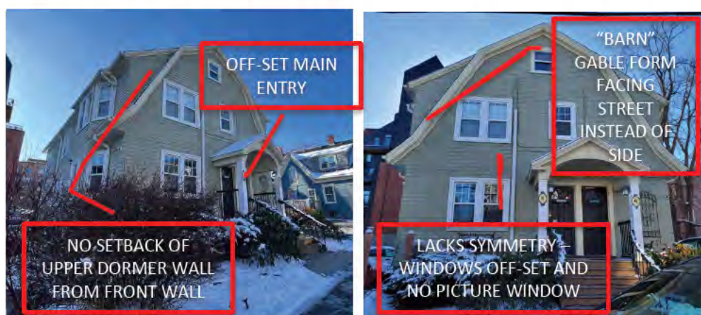
Figure 36a: Front components of 43-45 Dundas Street that detract from the style and overall design of a Dutch Colonial Revival house.
