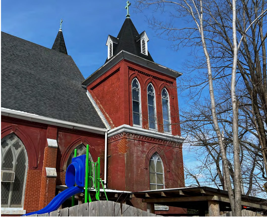
Figure 30c: South side tower
