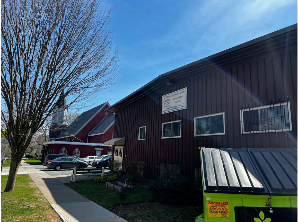
Figure 38: Context of 5540 Russell Street, St. Mark's Church in the background
