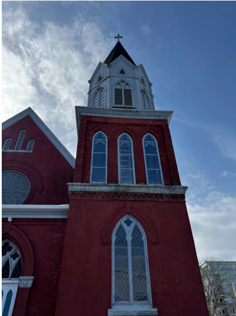
Figure 41g: St. Mark's Church, 5522 Russell Street (north tower)
