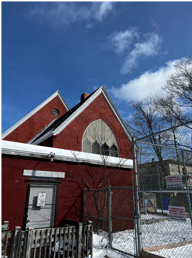
Figure 31c: Single-storey addition wrapping around the west side of 5522 Russell Street, with a single emergency exit door
