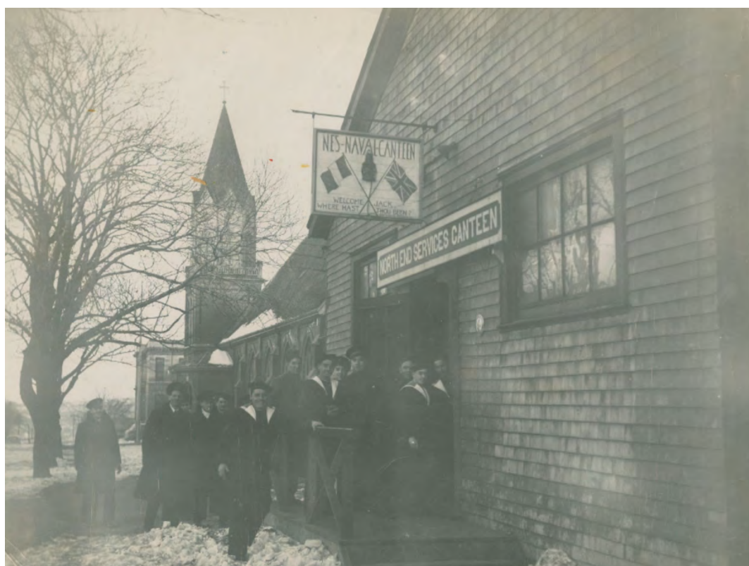
Figure 36: North End Services Canteen on Russell Street, behind St. Mark's Church, c. 1945
