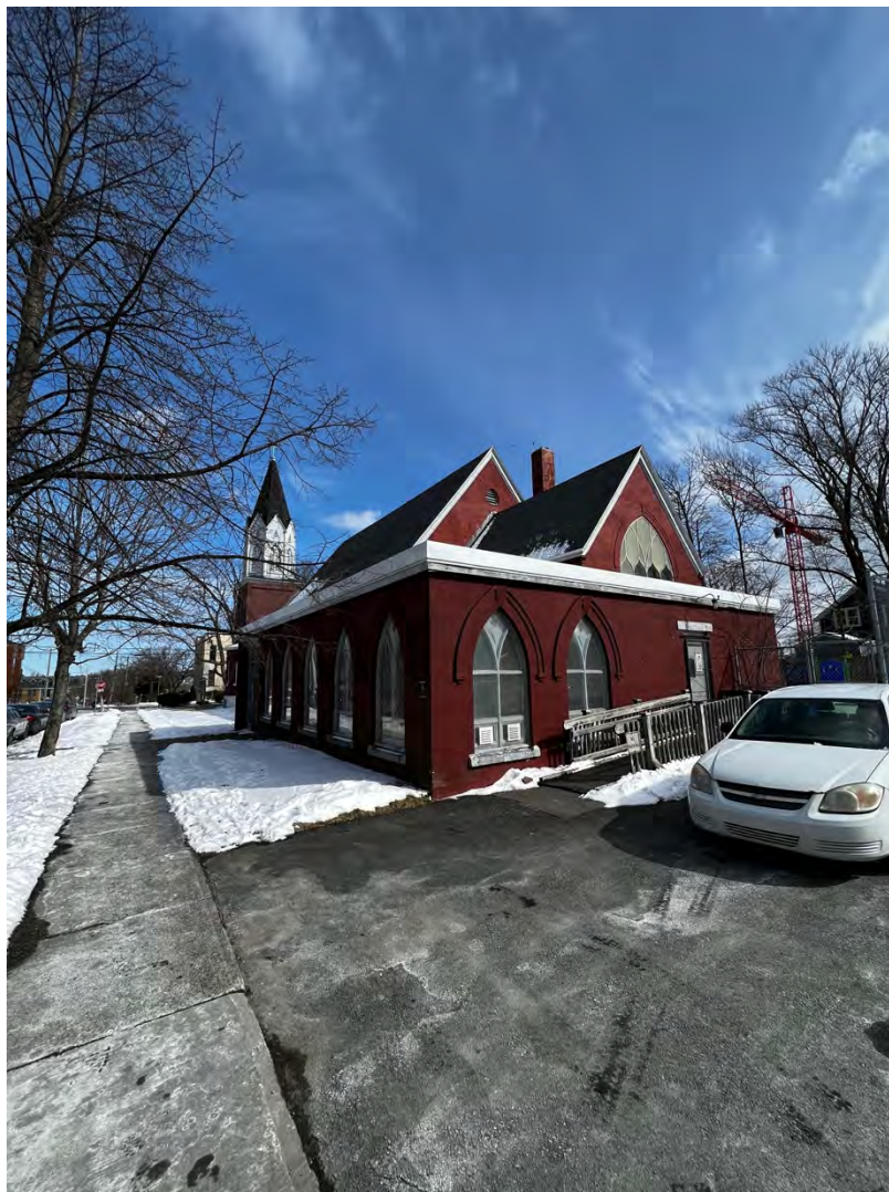
Figure 31a: Single-storey addition on the north side of 5522 Russell Street, as seen from Russell Street
