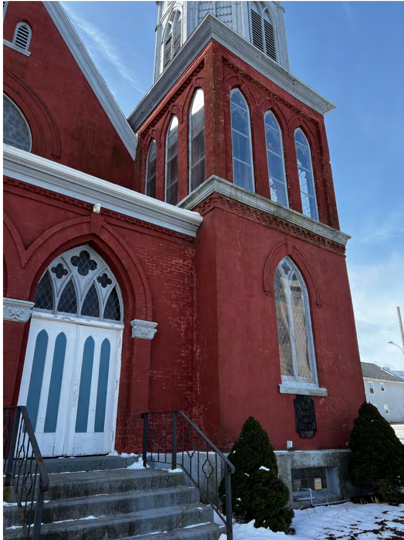
Figure 41f: St. Mark's Church, 5522 Russell Street (north tower)
