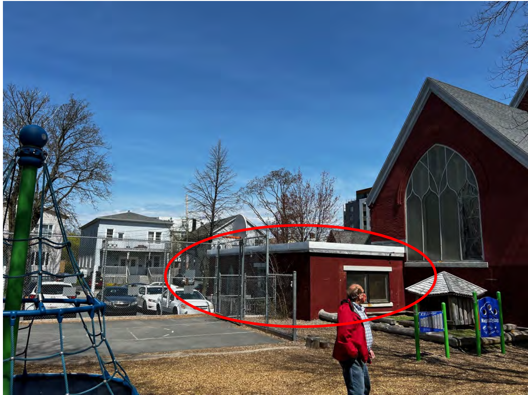
Figure 31b: Single-storey addition on the north side of 5522 Russell Street, seen from the rear and ending at the edge of the apse windows (circled)
