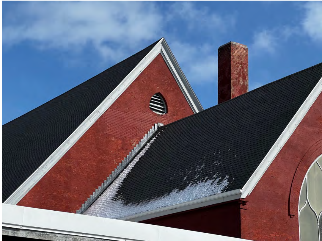
Figure 41m: St. Mark's Church, 5522 Russell Street (rear walls of main body and apse)
