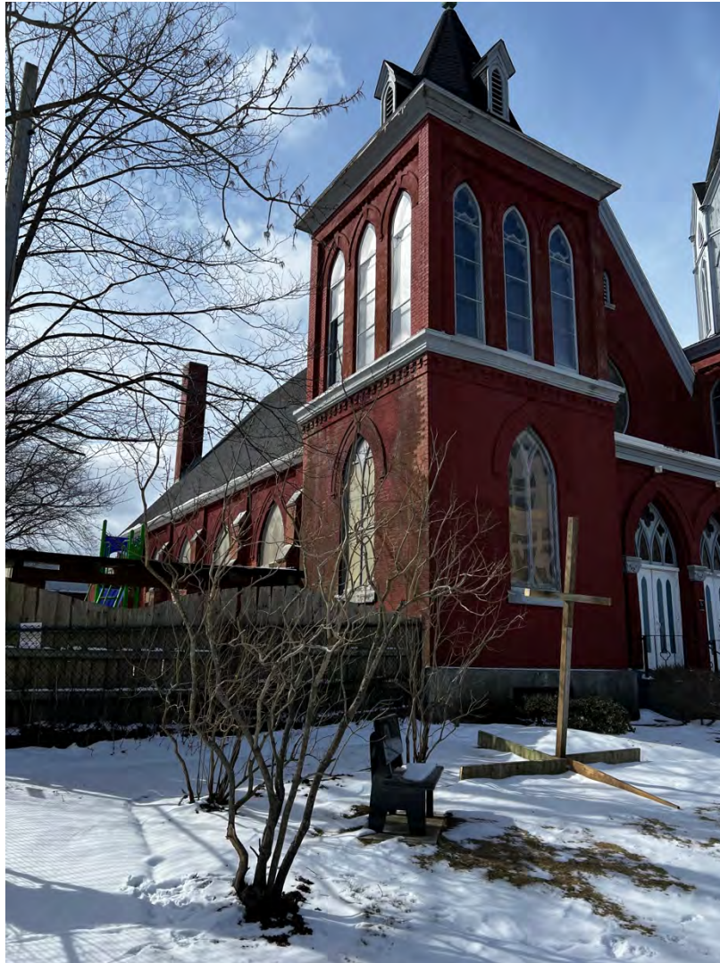
Figure 41c: St. Mark's Church, 5522 Russell Street (south tower)
