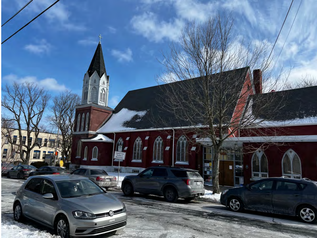
Figure 29b: Context of St. Mark's Church, 5522 Russell Street (seen from side, along Russell Street)
