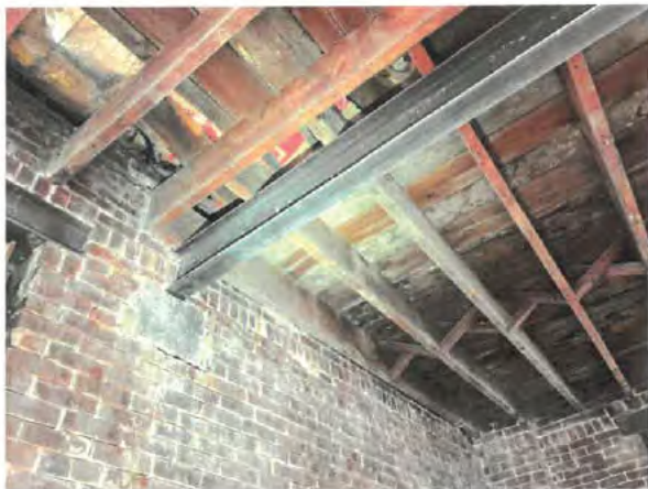
Photo No. 19 – Steel beam bearing at exterior wall.
