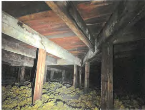
Photo No. 22 – View of attic space. Sloped roof support framing with props to ceiling joists below. Insulation on top of ceiling visible.
