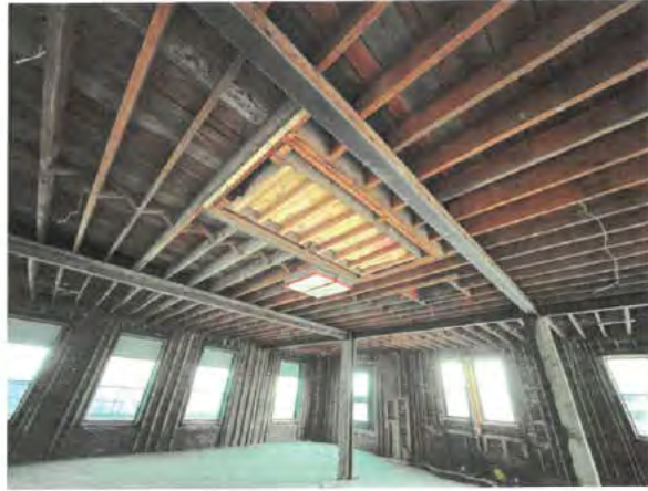
Photo No. 18 – Interior grid steel girders supporting roof. Note wood headers at former roof opening.
