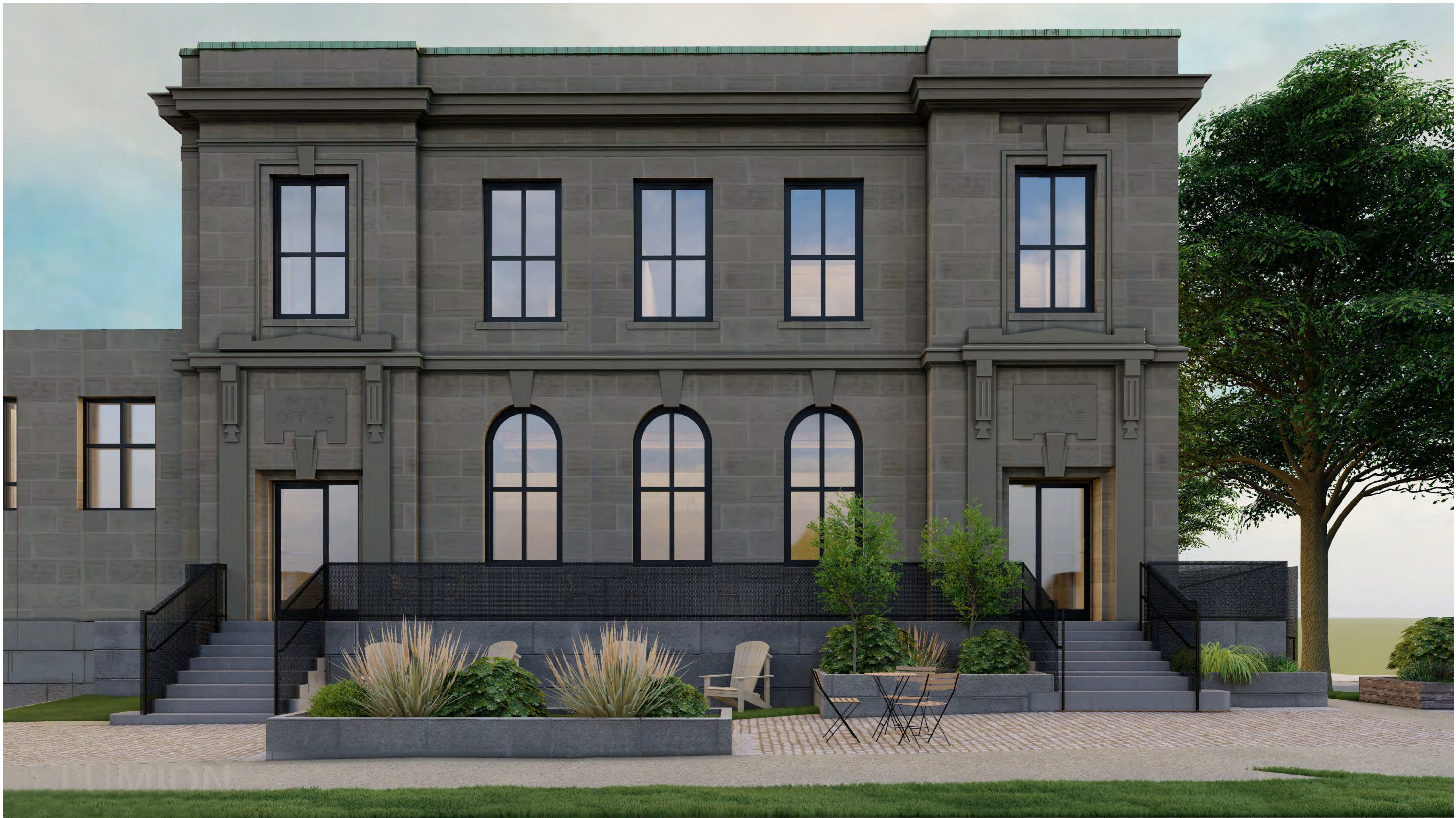
EAST ELEVATION (QUEEN STREET)
