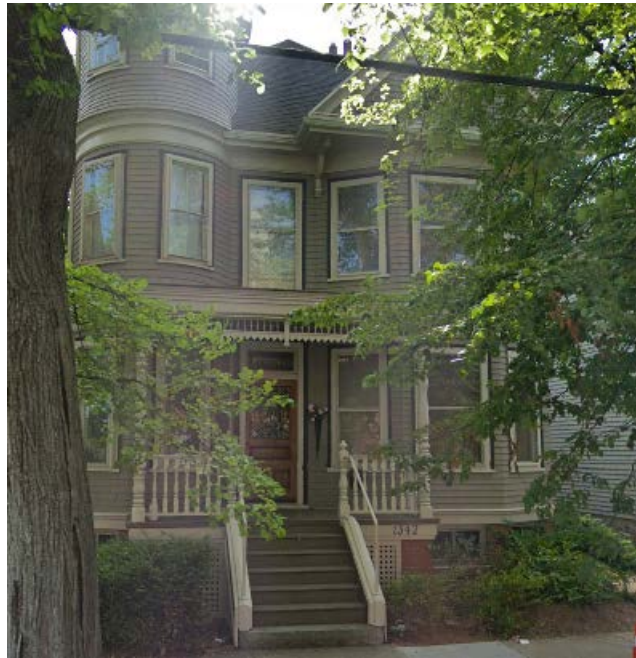
Figure 2: 1342 Robie Street in 2009 (Source: Google Maps)
