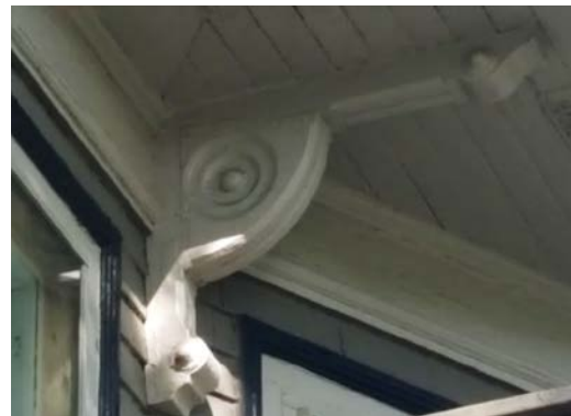
Figure 7: Console Under Eave (Source: Mia Rankin)
