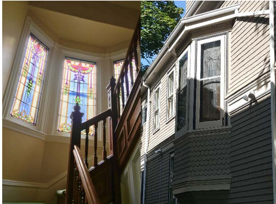
Figure 6: Interior Oriel Window; Exterior of Bay Window with Scalloped Shingles (Source: Mia Rankin)
