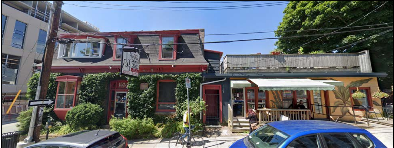
Figure 1: Second Empire style brick building with a one-storey addition at 1528-36 Brunswick Street at the corner of Doyle Street and Brunswick Street (Google Street View 2018)
