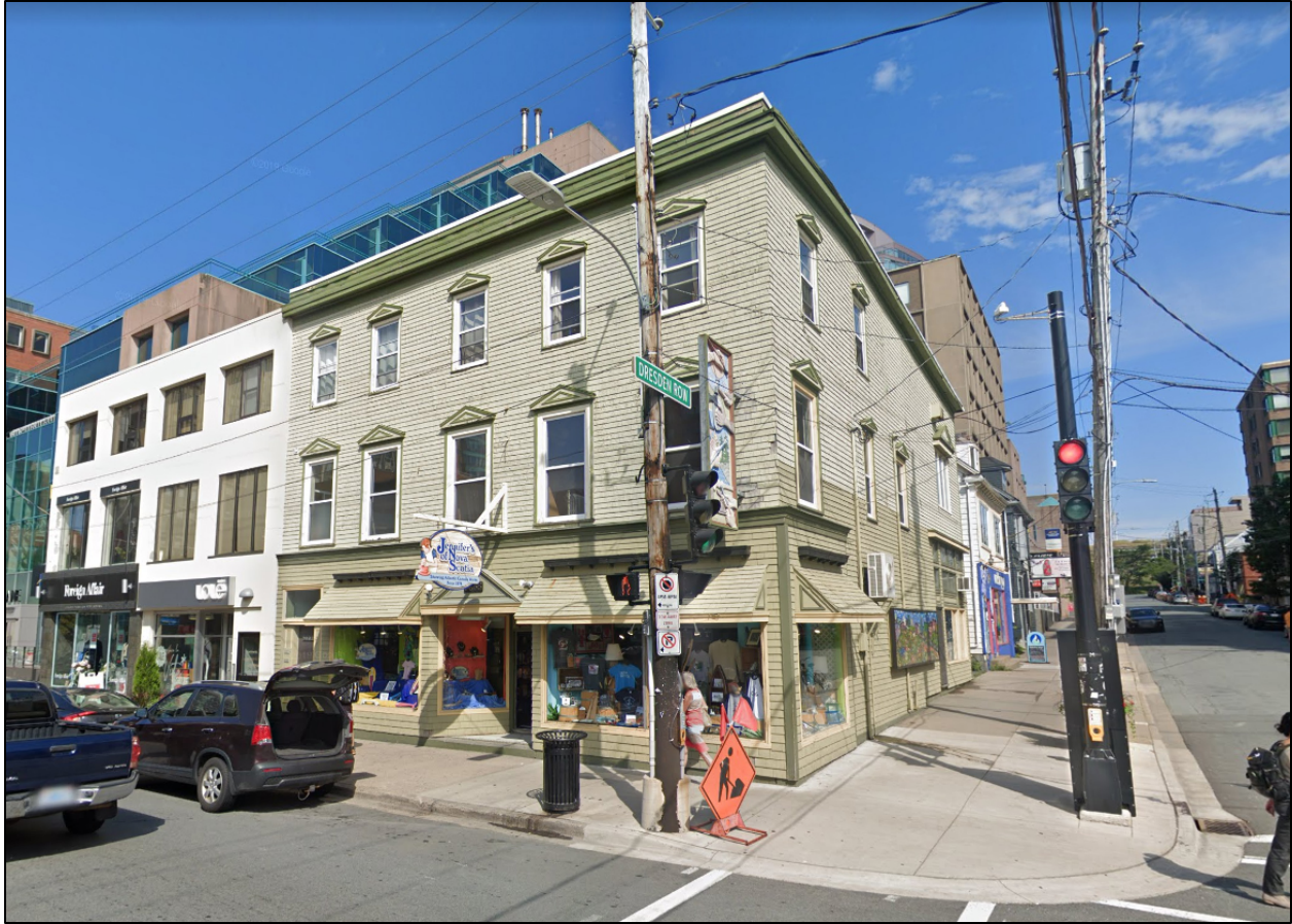
Figure 1: Originally a two-and-a-half storey Georgian-style residential building, the building at 5635-37 Spring Garden Road was converted to its present three-storey form when it was adapted for commercial uses c. 1920 (Google Street View 2018).
