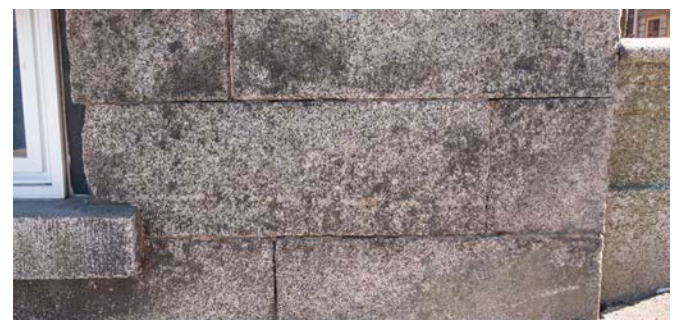
Figure 12. Existing Building Foundations
