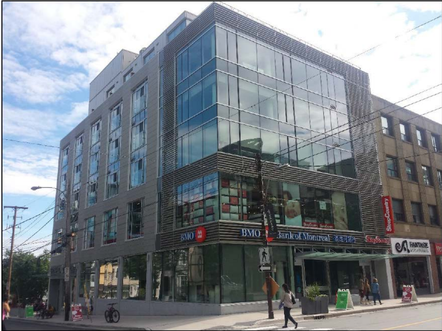
Photograph 1: Corner of Spring Garden Road and Birmingham Streets.
