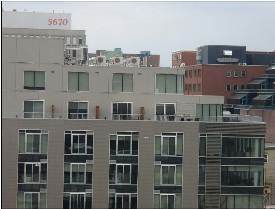
Photograph 6: Close-up view of upper floors and roof areas.
