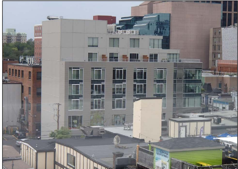
Photograph 5: View of upper floors and roof areas.
