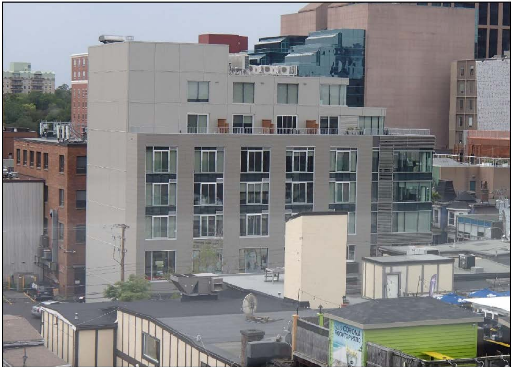
Photograph 5: View of upper floors and roof areas.
