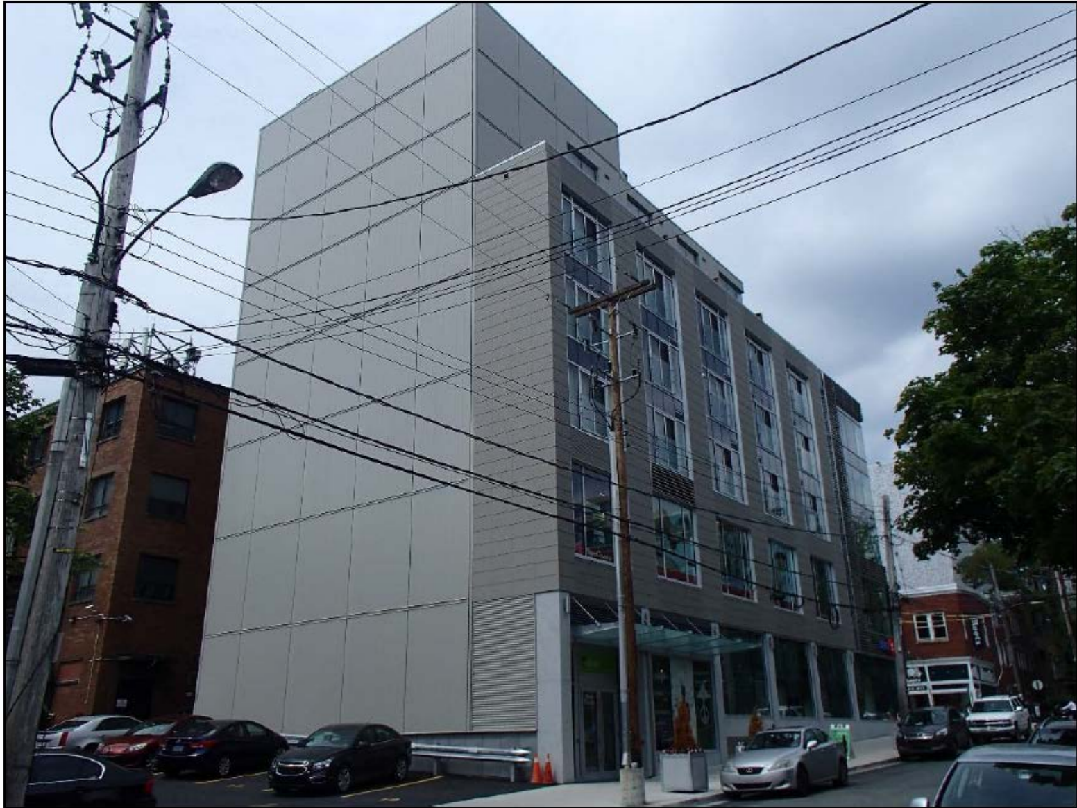
Photograph 2: Birmingham Street showing rear and side elevations.
