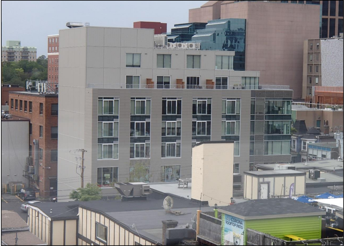
Photograph 5: View of upper floors and roof areas.
