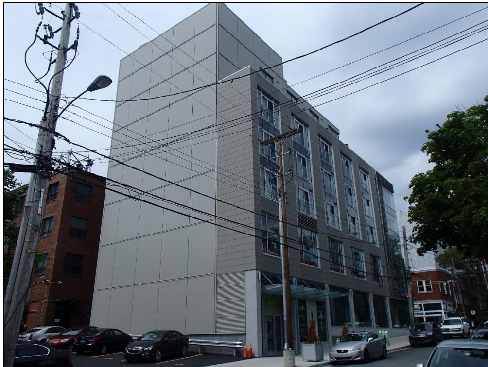
Photograph 2: Birmingham Street showing rear and side elevations.
