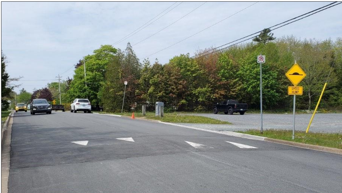
Speed hump located adjacent to existing driveway
