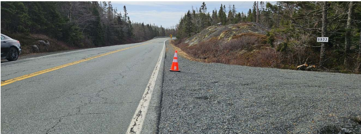
Prospect Road at Existing Driveway on right looking south
