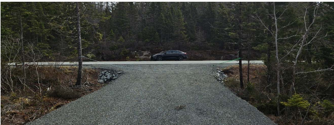
Existing Driveway to Prospect Road looking east
