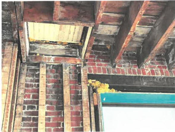
Photo No. 21 – Attic roof hatch at former Clock Tower location (South East).
