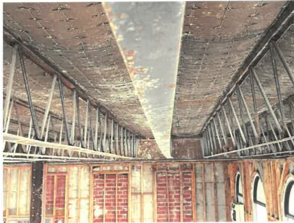
Photo No. 27 – Close view of 1947 roof joist.
