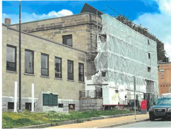
Photo No. 1 – View from Queen Street – South Elevation. Low roof area at left side will be demolished.
