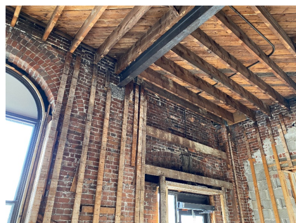
BMR Photo 4.4.F: Timber joists bearing on exterior masonry wall. Girder beam bearing on granite block (28 Feb 2022).
