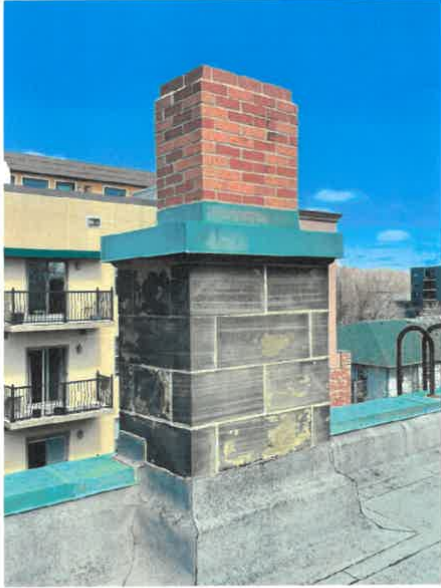
Photo No. 5 – Chimney in good condition.
