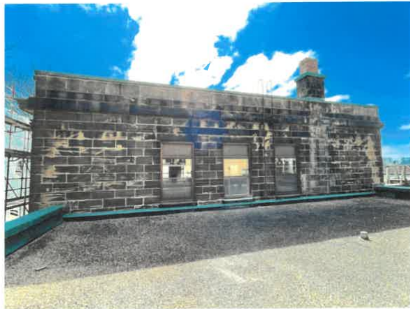
Photo No. 3 – North Elevation, original 1914 building, wall above 1947 roof.
