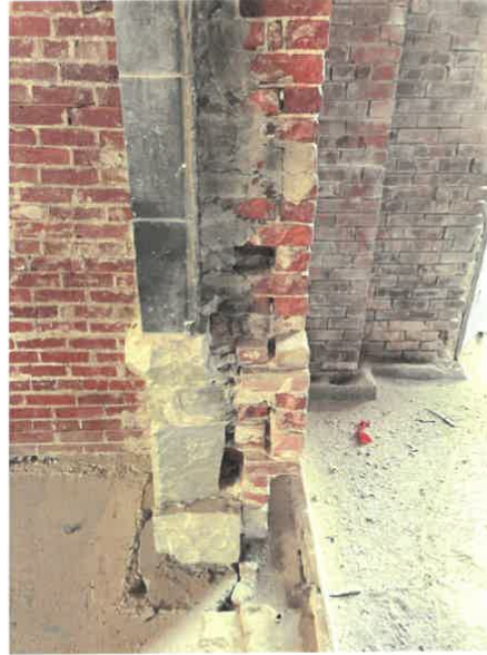
Photo No. 14 – Opening through existing wall with window sill cut out. Sandstone facing with three wythe brick back up wall.
