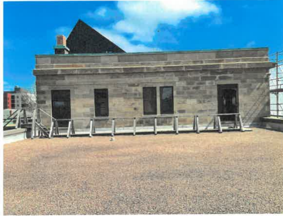
Photo No. 2 – West Elevation above 1961 addition roof.
