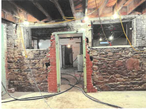
Photo No. 25 – Pier removal at door opening.
