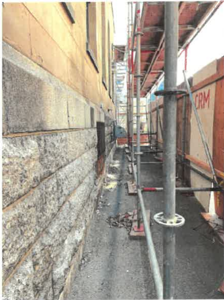
Photo No. 7 – Foundation at grade with granite facing and sandstone above.
