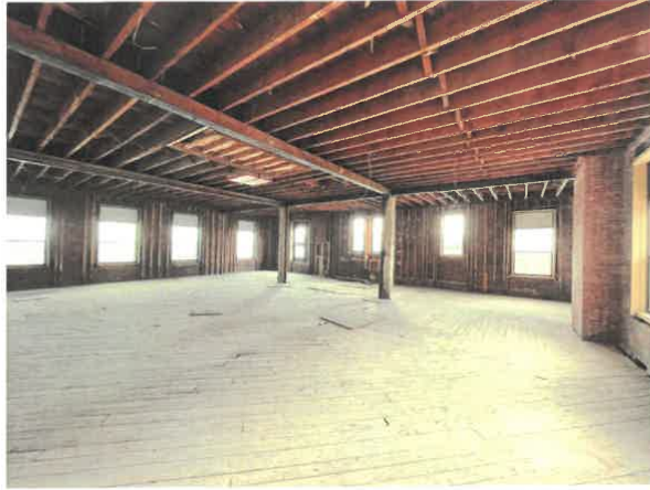
Photo No. 17 – Second floor of 1914 block with ceiling and roof support joists visible. Steel girders and concrete encased columns visible.
