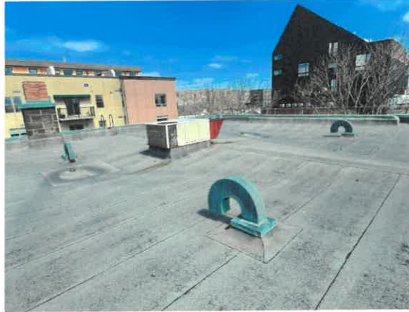
Photo No. 6 – Upper roof (1914) with slopes to drains.
