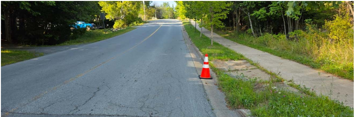
229 Holland Road at proposed new site access on right looking north
