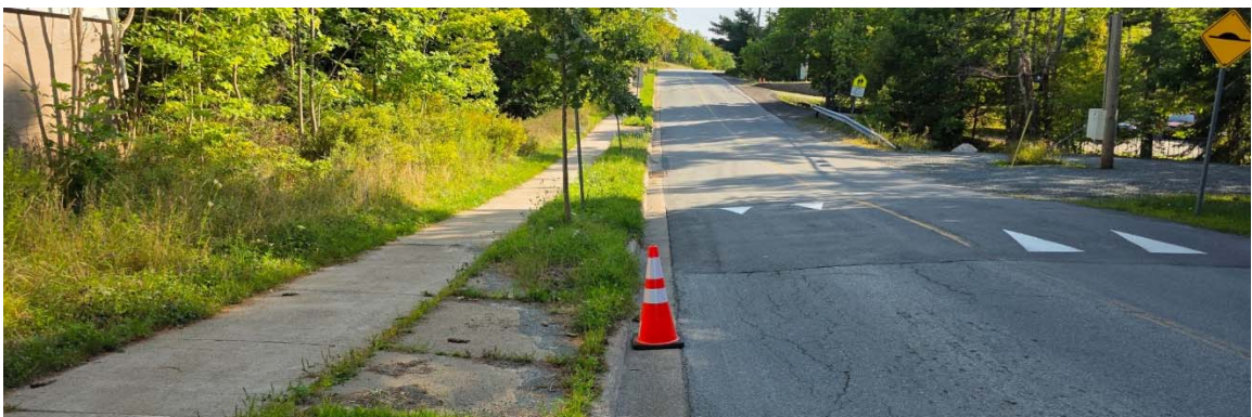
229 Holland Road at proposed new site access on left looking south
