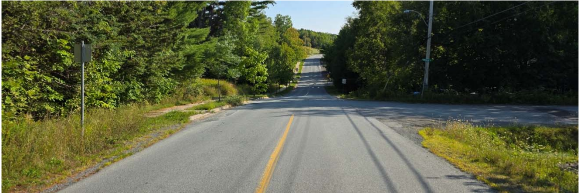
Holland Road at Brook Street looking south
