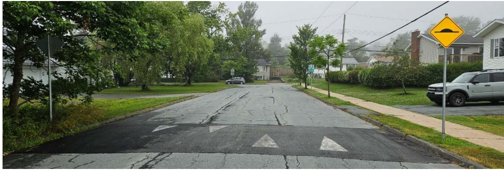
Evergreen Drive at Poplar Drive looking west (with traffic calming speed hump)
