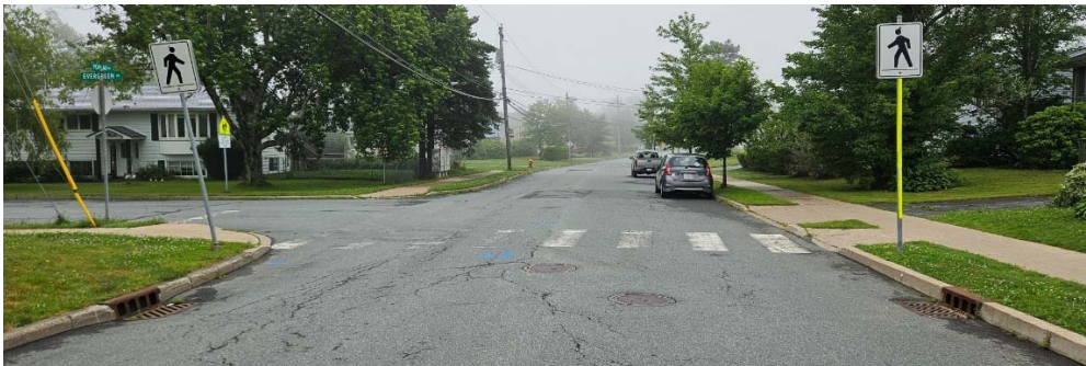
Evergreen Drive at Poplar Drive looking south (marked crosswalk)
