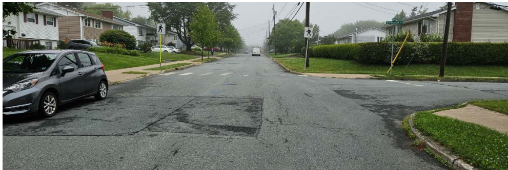
Evergreen Drive at Poplar Drive looking north (marked crosswalk)
