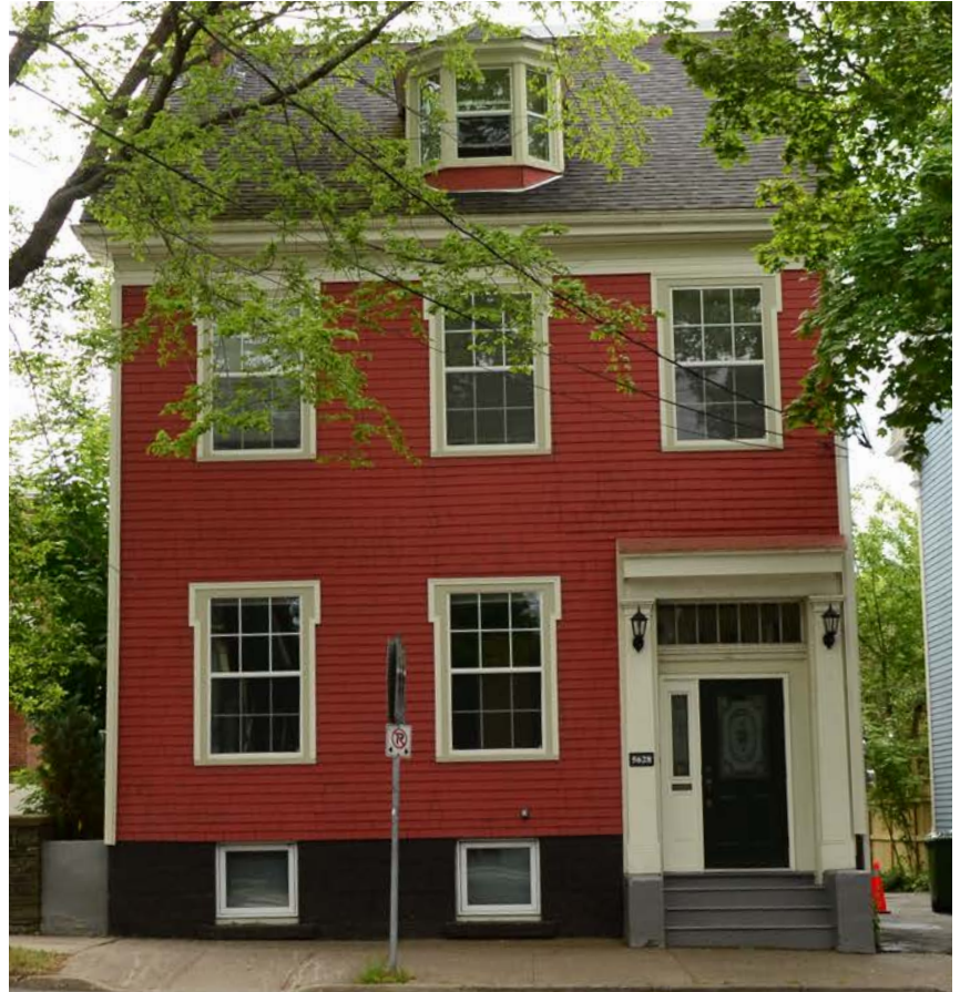
Home showing an example of a Georgian style fenestration pattern, including a street-oriented Scottish Dormer.
