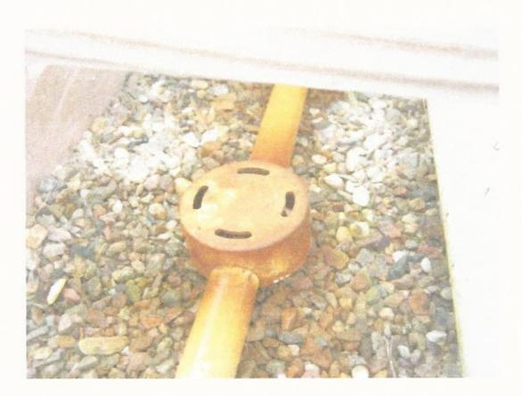
Figure 2. Iron oxide coating on pipes and pea gravel in the ETI RSF
