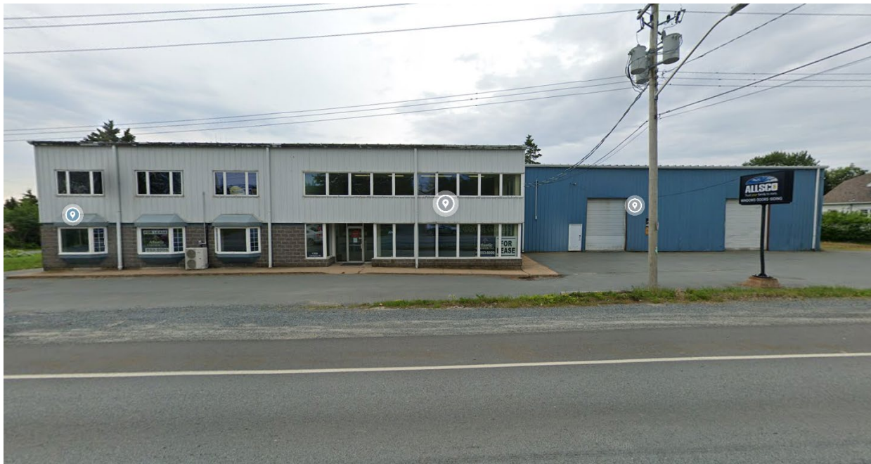
Street view of the subject site
