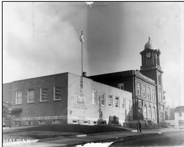
Figure 12: Photograph of the Dartmouth Federal Building and Post Office, 1960s (Source: HRM Archives, 2018).
