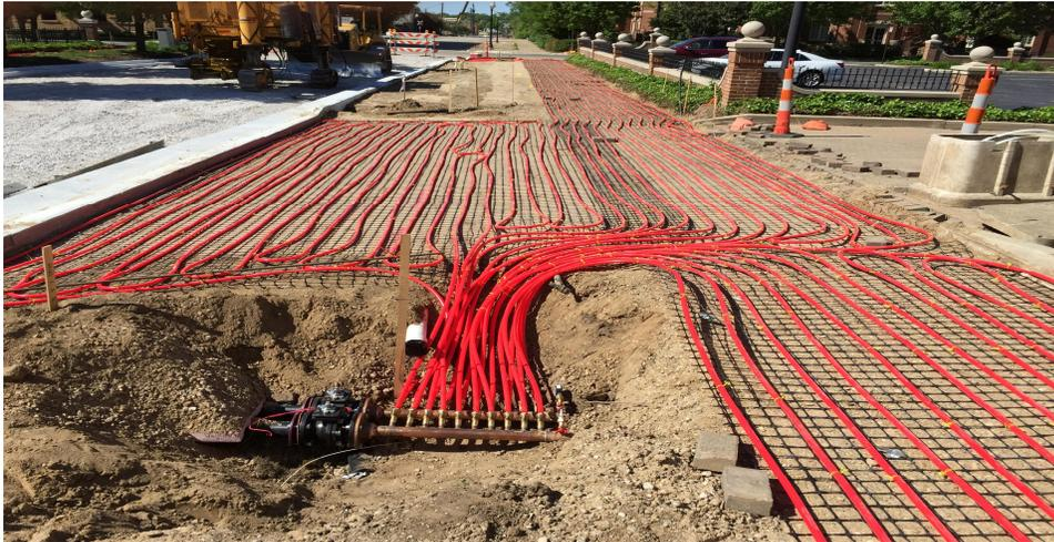
Typical Snowmelt Tubing Manifold
