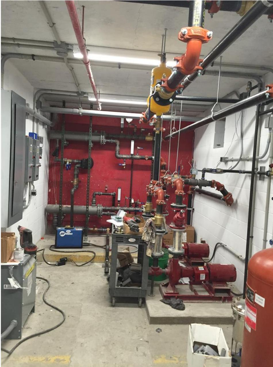
Typical snowmelt system mechanical room with heat exchangers and pumps
