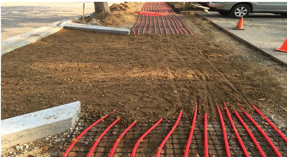
Example of Snowmelt Tubing Covered with Gravel Prior to Paving
