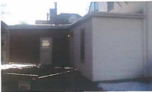
Figure 5: Rear of east addition
