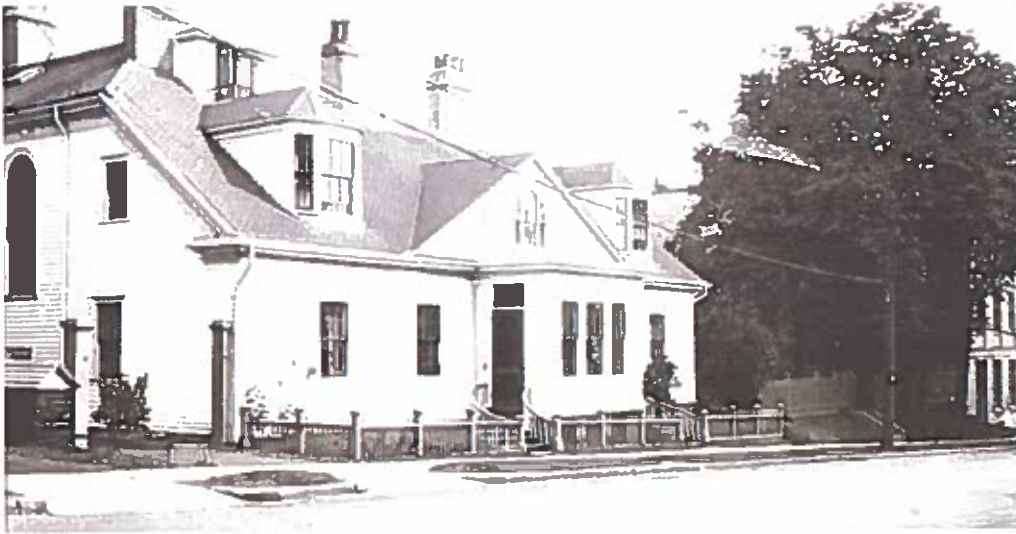
Figure 19: early view looking east 13
