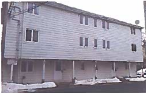
Figure 9: Old Carriage House - South Elevation
