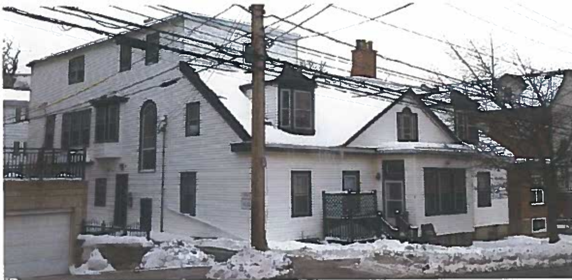
Figure 2: From the Southwest showing rear wing with third floor addition
