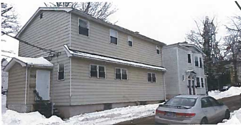
Figure 11: 5230 Harvey Street (foreground, 5240-46 background)
