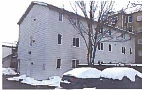
Figure 10: Old Carriage House - From the north-east
