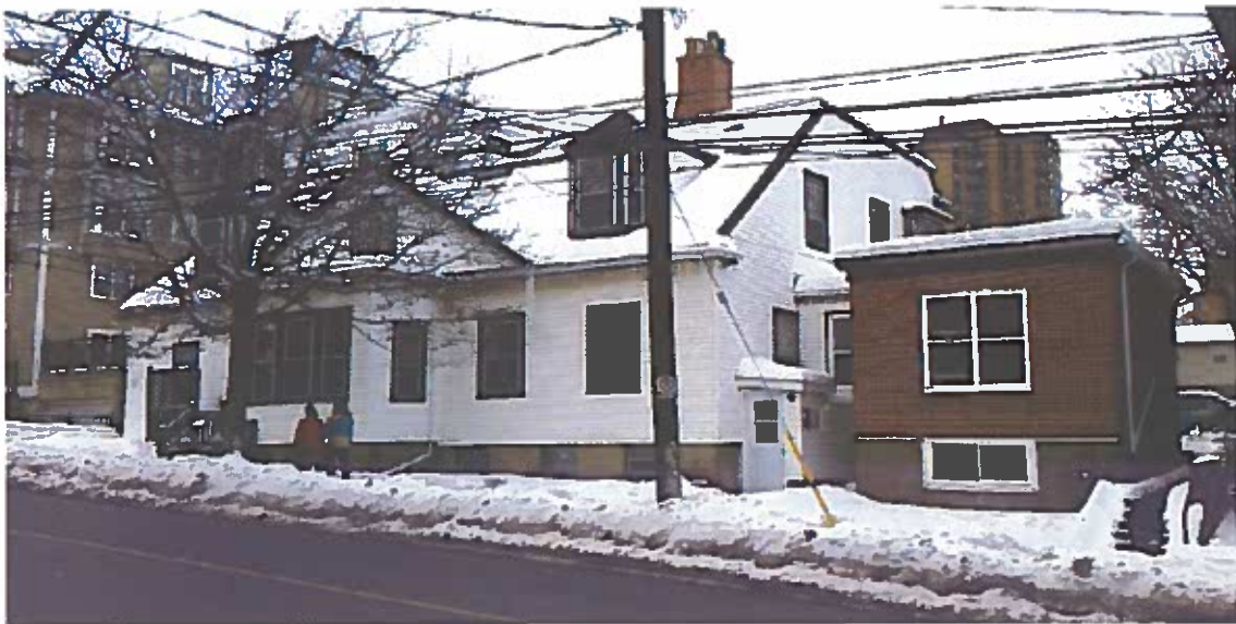
Figure 3: From the Southeast showing later one storey additions
