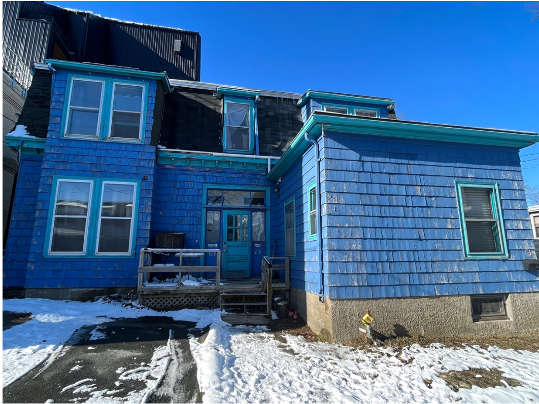
Figure 28a: Alexander and Maude MacKay Residence, 61 Queen Street – front, with later office extension shown on the right
