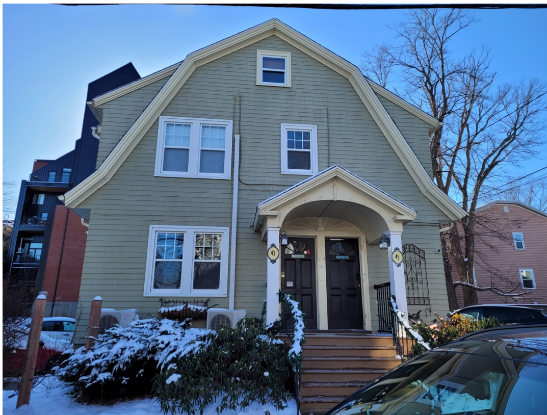
Figure 33a: 43-45 Dundas Street, front
