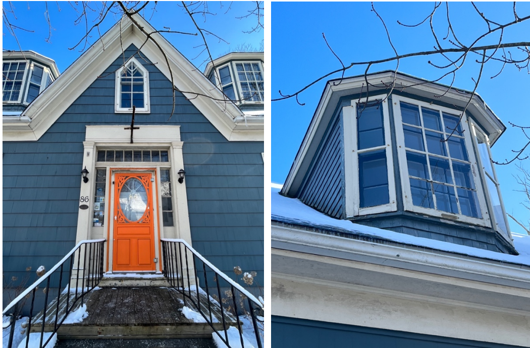
Figure 22d: George and Mary Shiels Residence, 86 Ochterloney Street – Front detail including entry, sidelights and transom, and central-set gable; upper window detail – Scottish dormers
