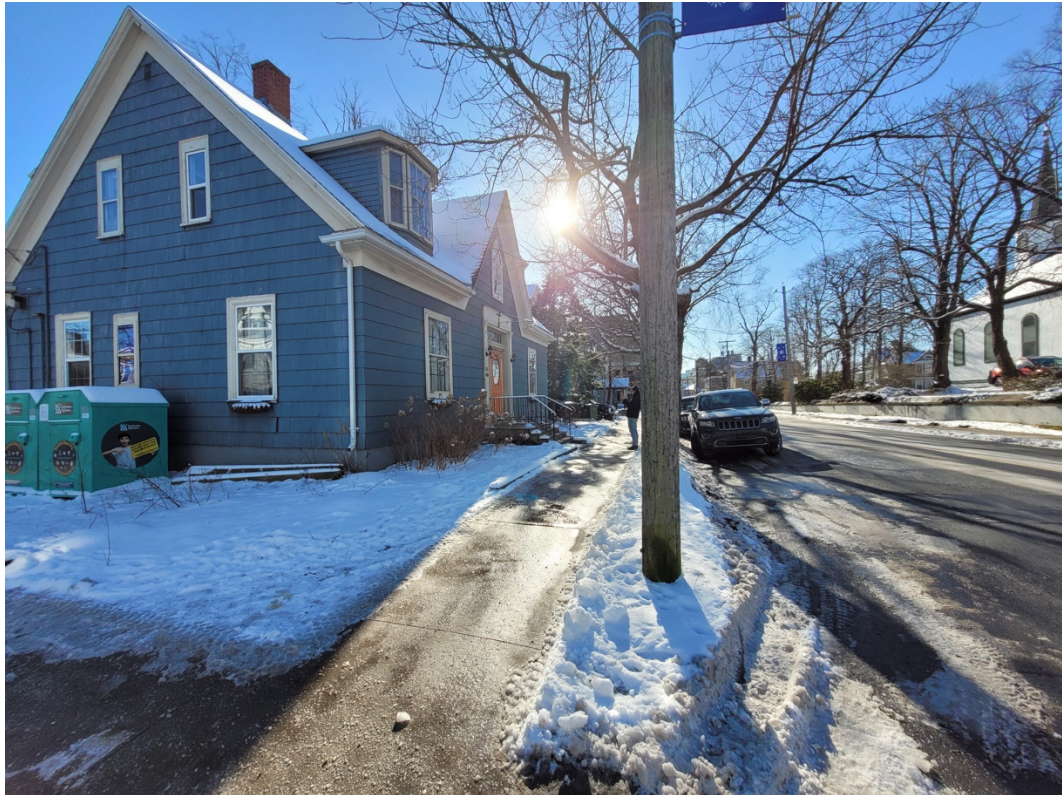
Figure 21b: Context of 86 Ochterloney Street (front, looking southwest along Ochterloney Street) – neighbouring Christ Church on the far right
