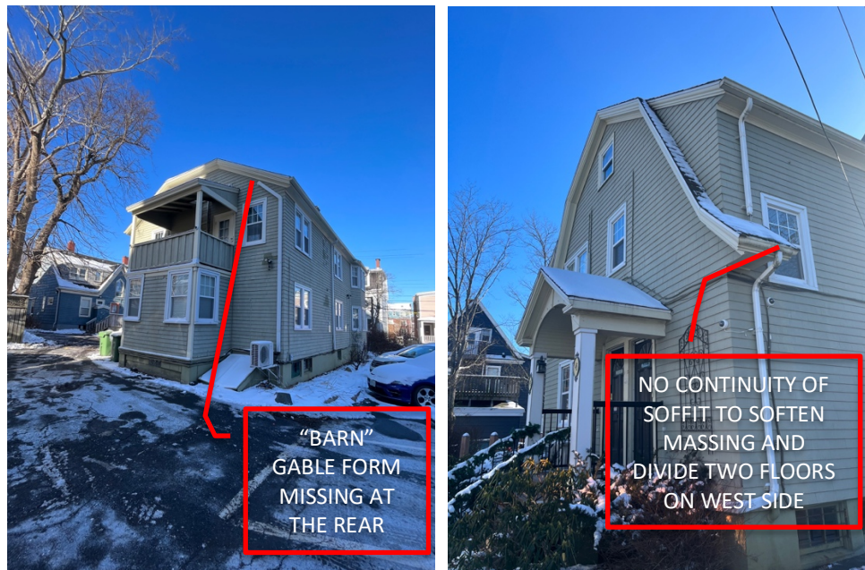
Figure 35: Front and rear components of 43-45 Dundas Street that detract from the style and overall design of a Dutch Colonial Revival house.
