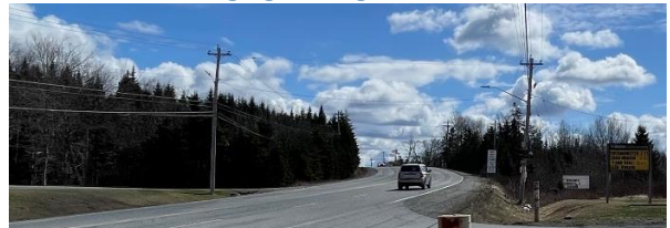
Photo 4: Looking right along Trunk 7 from Access 2
