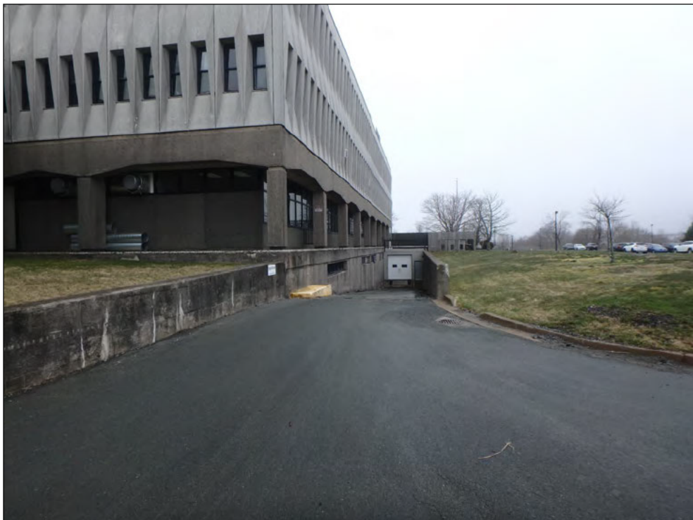
Plate 15: Underground receiving dock for the west-most building of the Research Drive complex, looking northwest.
