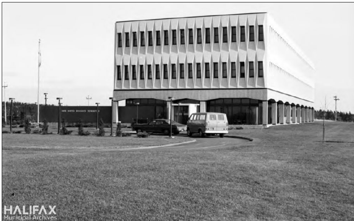
Figure 4-16: Photo of the Nova Scotia Research Foundation ca. 1970, looking east. 110
