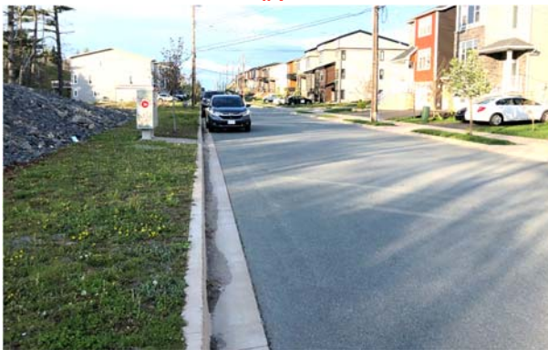
Photo 6 – Looking East (to the left) on Fleetview Drive from Approximate location of Future Driveway #2
